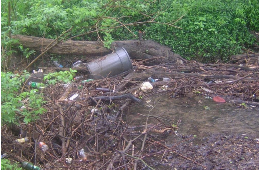
Figure 20 – Accumulated trash and debris in sinkhole in Big Spring Park
