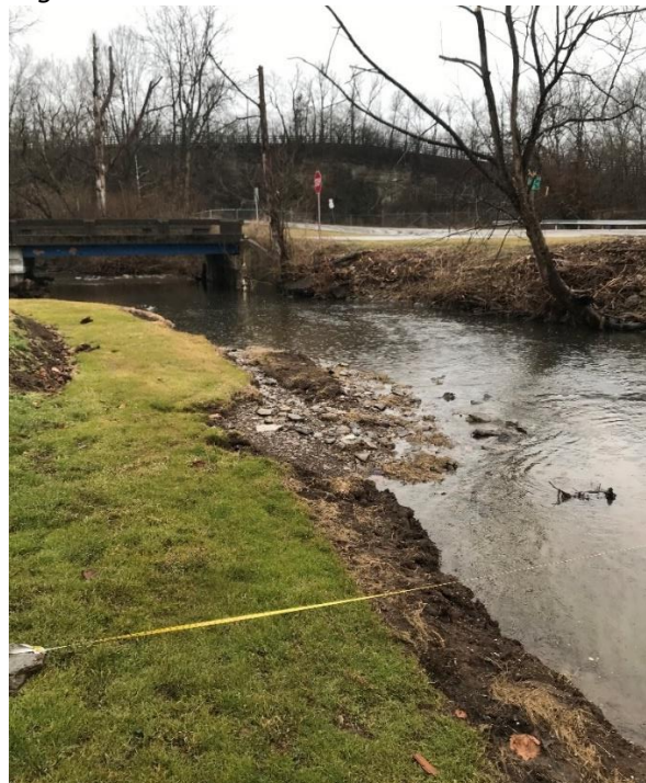
Downstream view from left bank on February 2 showing erosion of unprotected soil from bank
